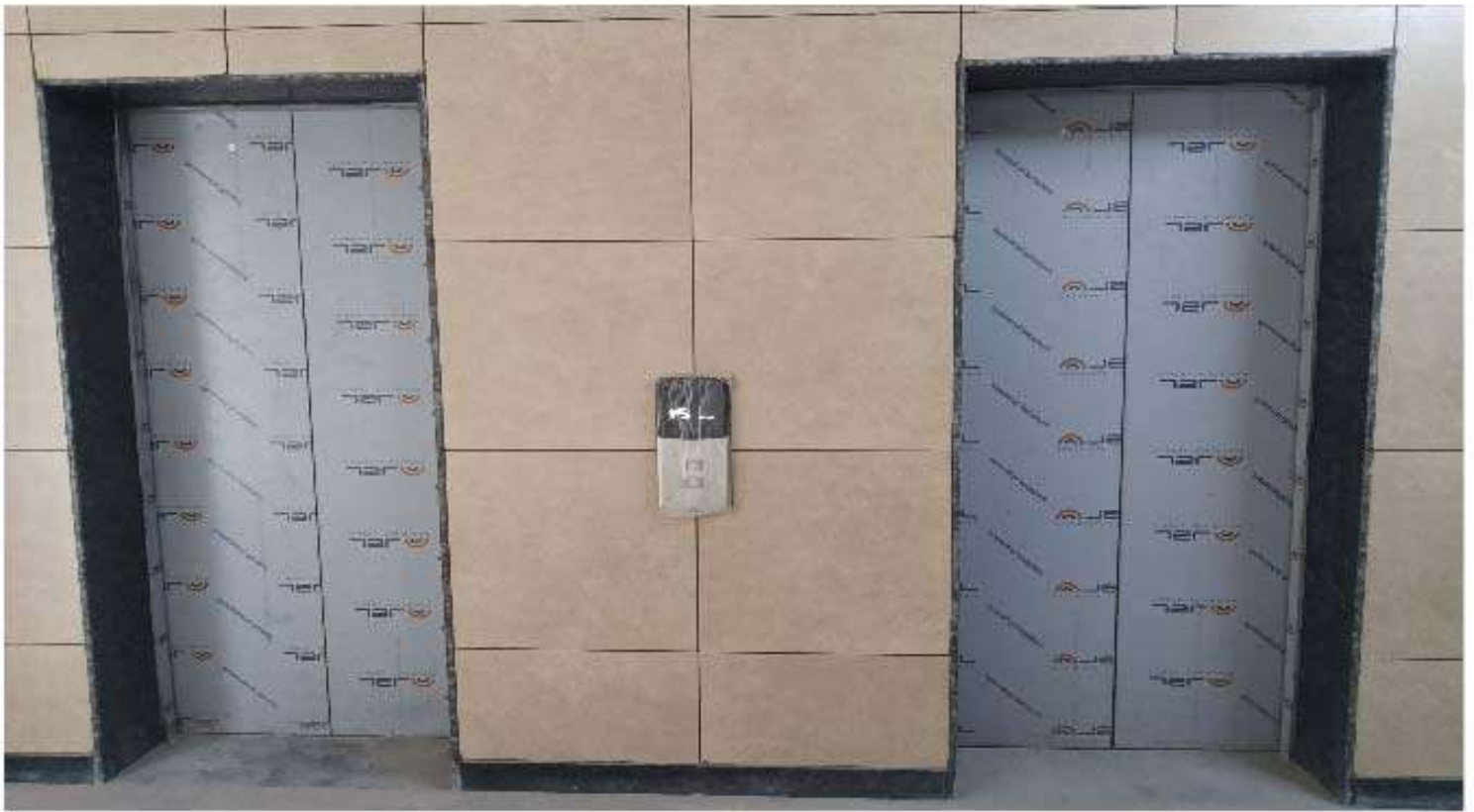
BLOCK 3 LIFT INSTALLATION COMPLETED
